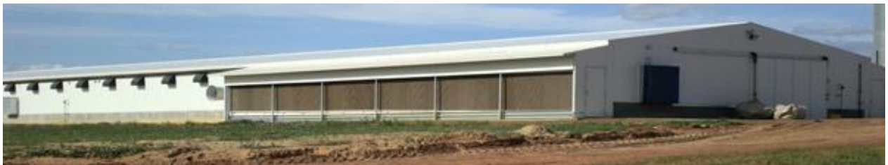
Mechanically ventilated broiler house with cooling pads
