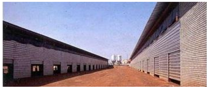
Floors of high-rise layer houses are elevated with openings for droppings to fall down to the ground.
